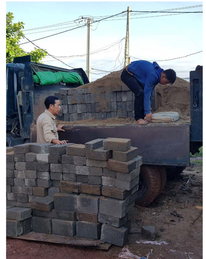
Toilet construction process / Quang Tri Province
